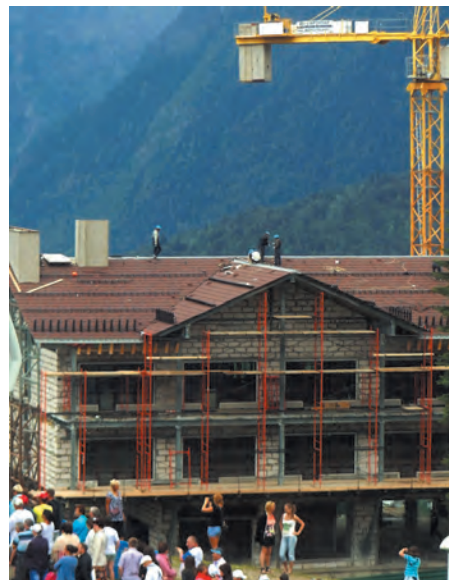
Source: Picture made by Rut Perez-Studer at Olympic construction site, Russia, 2012
